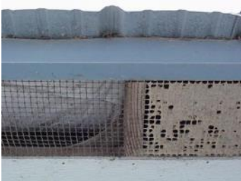
Soffits clean and clear?
